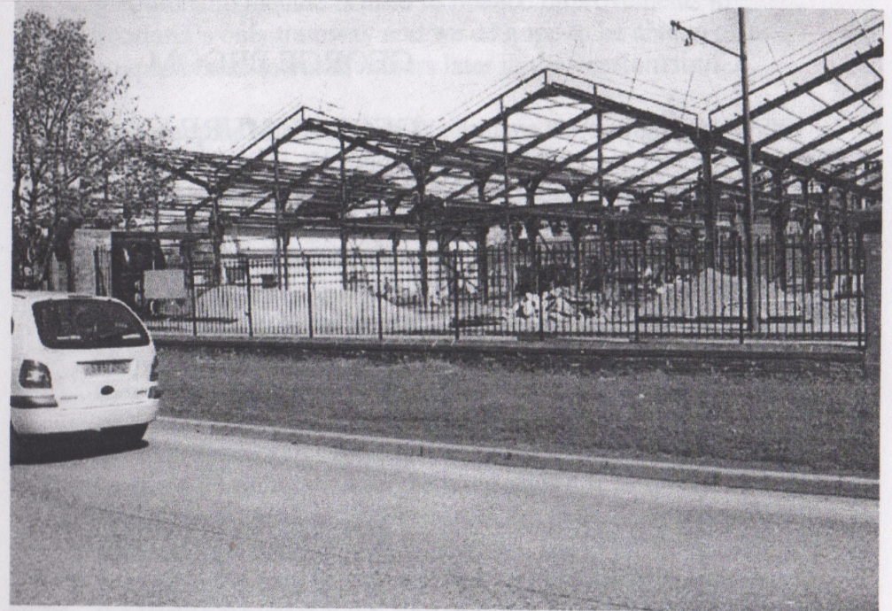
Work progressing on the Main Building
